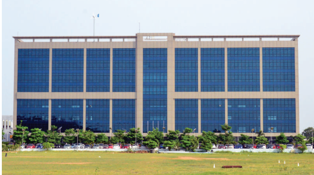
Intellect Design Arena Head Office, Chennai
